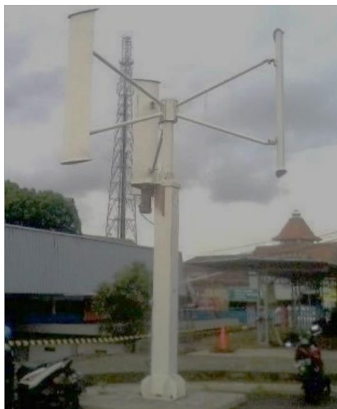
Gambar 2.7 Turbin Angin tipe Darrieus Sumber: ( Anis Fadila, 2020 )
