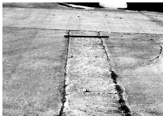
Gambar 2.10. Kerusakan Patching Large & Utility
