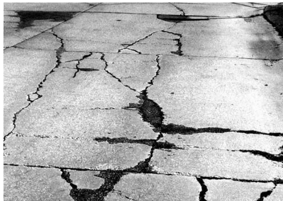
Gambar 2.4. Kerusakan Divided Slab
