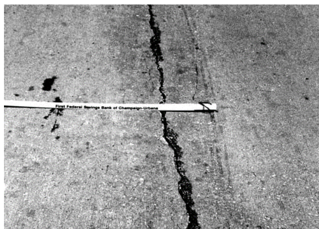
Gambar 2.9. Kerusakan Linear Cracking
