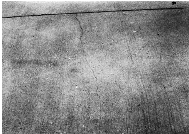
Gambar 2.18. Kerusakan Shrinkage Crack
