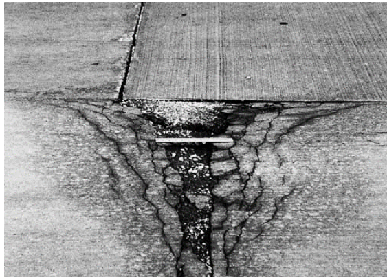
Gambar 2.5. Kerusakan Durability Cracking “D”
