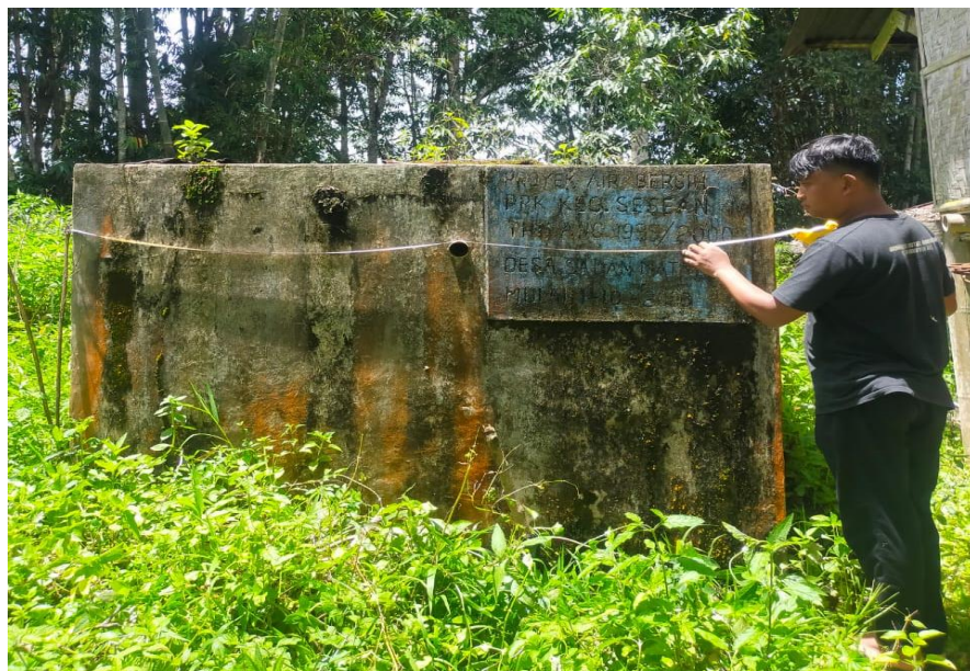
Pengukuran Bak Reservoir
