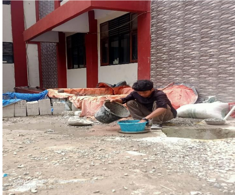
Proses Pengujian Kadar Lumpur Agregat
